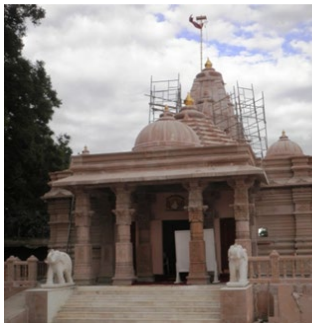
Completion of the Shikharbandh Derasar
